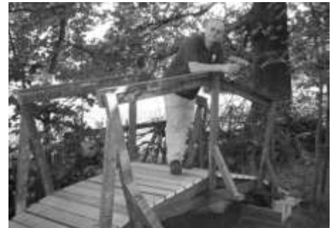
Phil on the bridge over the stream that drains the moat. Phil built this bridge as a "kit of parts", which was then assembled on site with help from members of the Yorkshire Area Group of the 16mm Association
